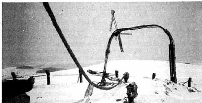
70MHz beacon GB3BUX after suffering some heavy weather
